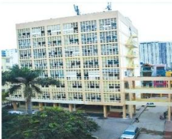
Repair and renovation of A18, Institute of Chemistry
