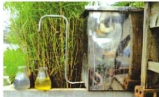
Treatment technology of wastewater containing Cr, Ni by combining sawdust with aquatic plants at pilot scale, capacity of 50 m3/ day
