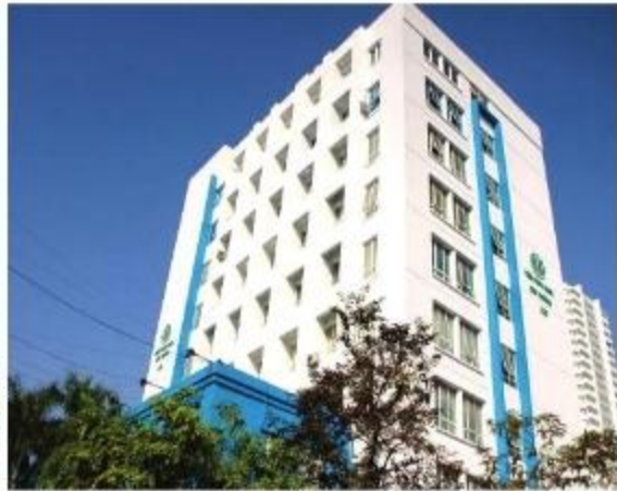
Renovation and additional storeys of Institute of Environmental Technology
