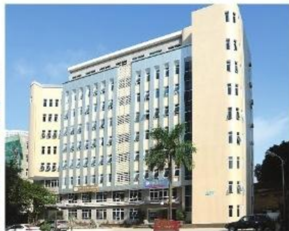
Renovation of A27 Building
